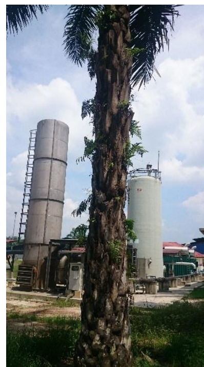
Havys Oil Mill Biorefinery in Malaysia
