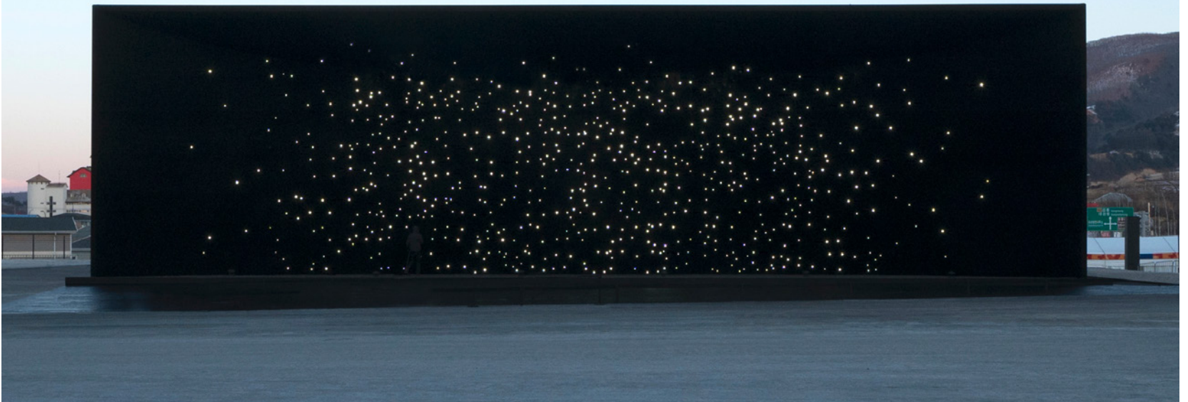
The Hyundai Pavilion at the 2018 Winter Olympics used Vantablack™ to create a striking visual effect of stars appearing to float in mid-air.
